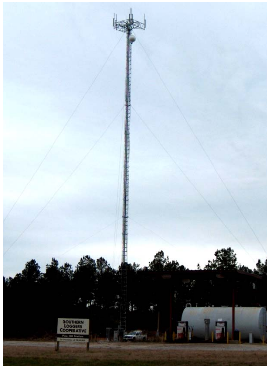
Pine Belt Wireless' Yellow Bluff Tower
